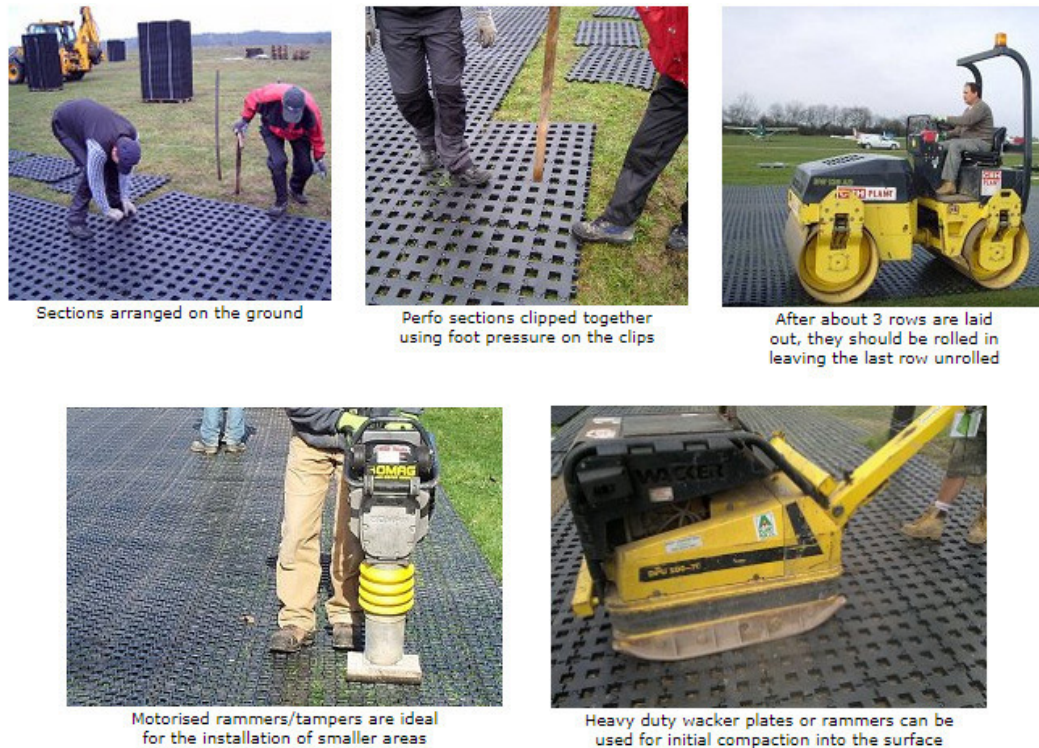
Fig. 9: Typical installation of reinforced-grass tiles (Perfo® Interlocking Ground Reinforcement)
