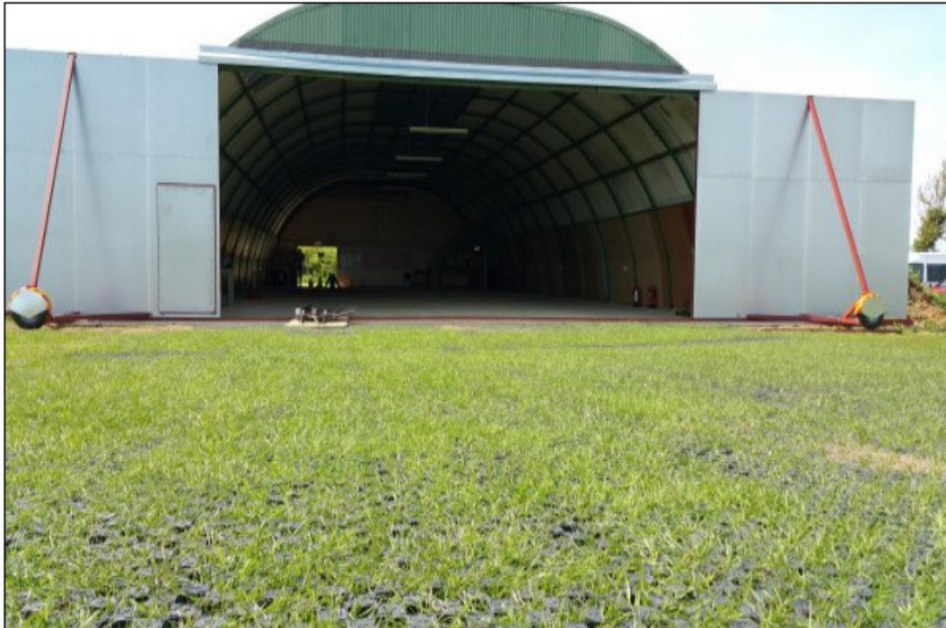
Fig. 8: Typical installation of reinforced-grass tiles (Perfo® Interlocking Ground Reinforcement)
